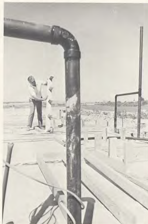
Warren Wyman, Rancho Santa Fe builder, lends a hand on early steps in one of the five houses he has under construction in the Isla Verde section at Lomas Santa Fe.
