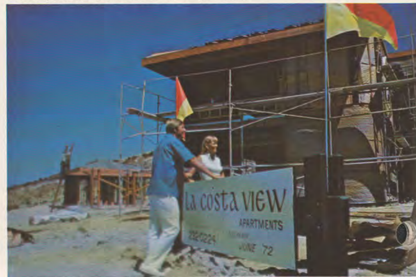
The couple look over La Costa View apartments—
