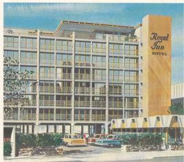
ROYAL INN HOTEL OF SAN FRANCISCO, CALIFORNIA. OPEN DECEMBER, 1968. Includes a Jolly King Restaurant.
