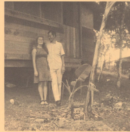
Mr. and Mrs. Robert Pitt beside the wooden frame home which they built with their own hands.
