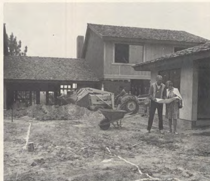
A special feature of the condominiums is absolute privacy. Chalk marks in the photograph above indicate the line of the five foot wall that will enclose the patio, screening it from the next unit. In the background is a nearly completed 2-story plan.
