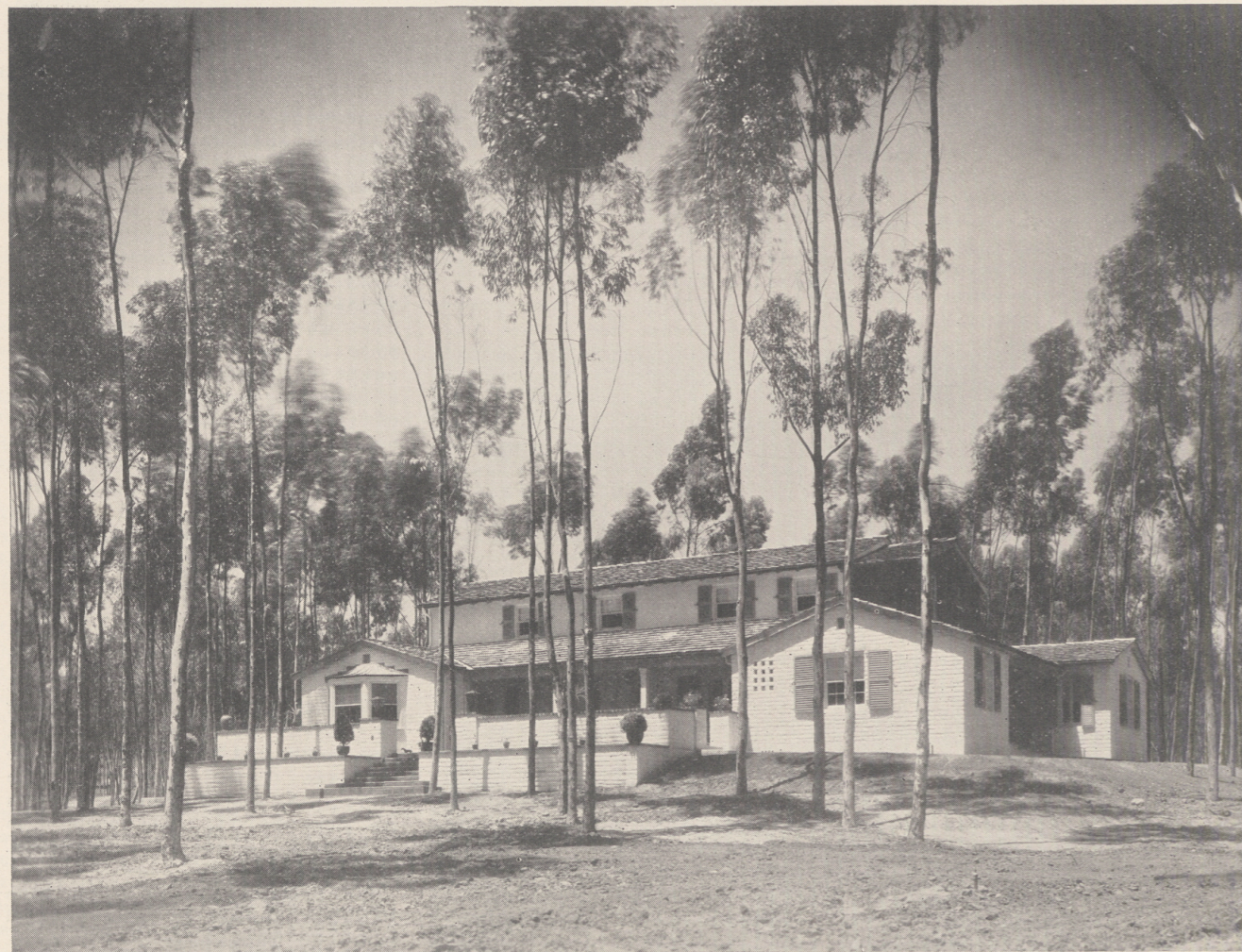
Resting serenely on its knoll in a forest of stately eucalyptus trees, the Gilbert home truly fits its environment. Its simple beauty is much commented upon.
