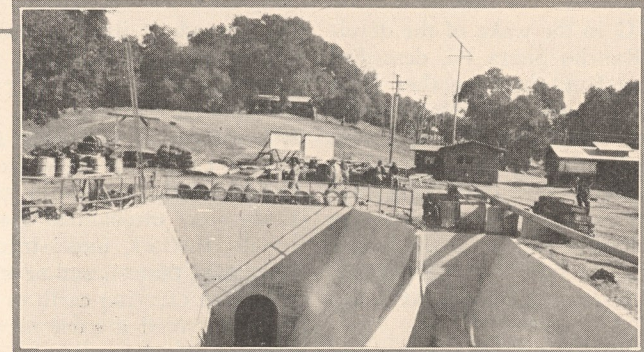
Here is shown excavation work attendant on the construction of the Henshaw Dam spillway
