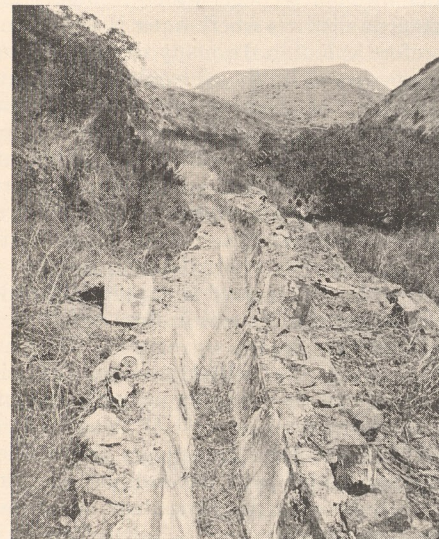
This conduit, about five miles in length, conducted the water from the dam to the site of the Mission
