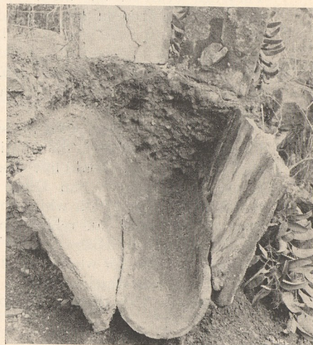
Here the structure of the conduit is shown. Many of the flat units now serve as flooring in "Ramona's Home," Old Town, San Diego
