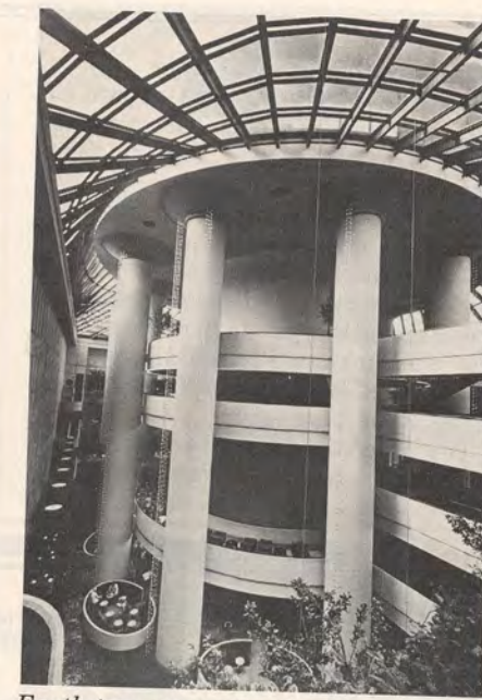
Earth-tone concrete columns rise seven stories out of a half-acre lake to the skylighted roof of the lobby in the new Peachtree Plaza Hotel.
