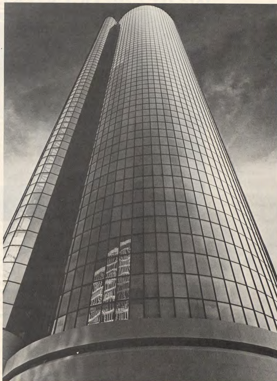
The soaring guest-room tower of the new 70-story Peachtree Plaza. Glass-enclosed elevators to the hotel's revolving restaurant and cocktail lounge are located in the tube-like exterior shaft (left).
