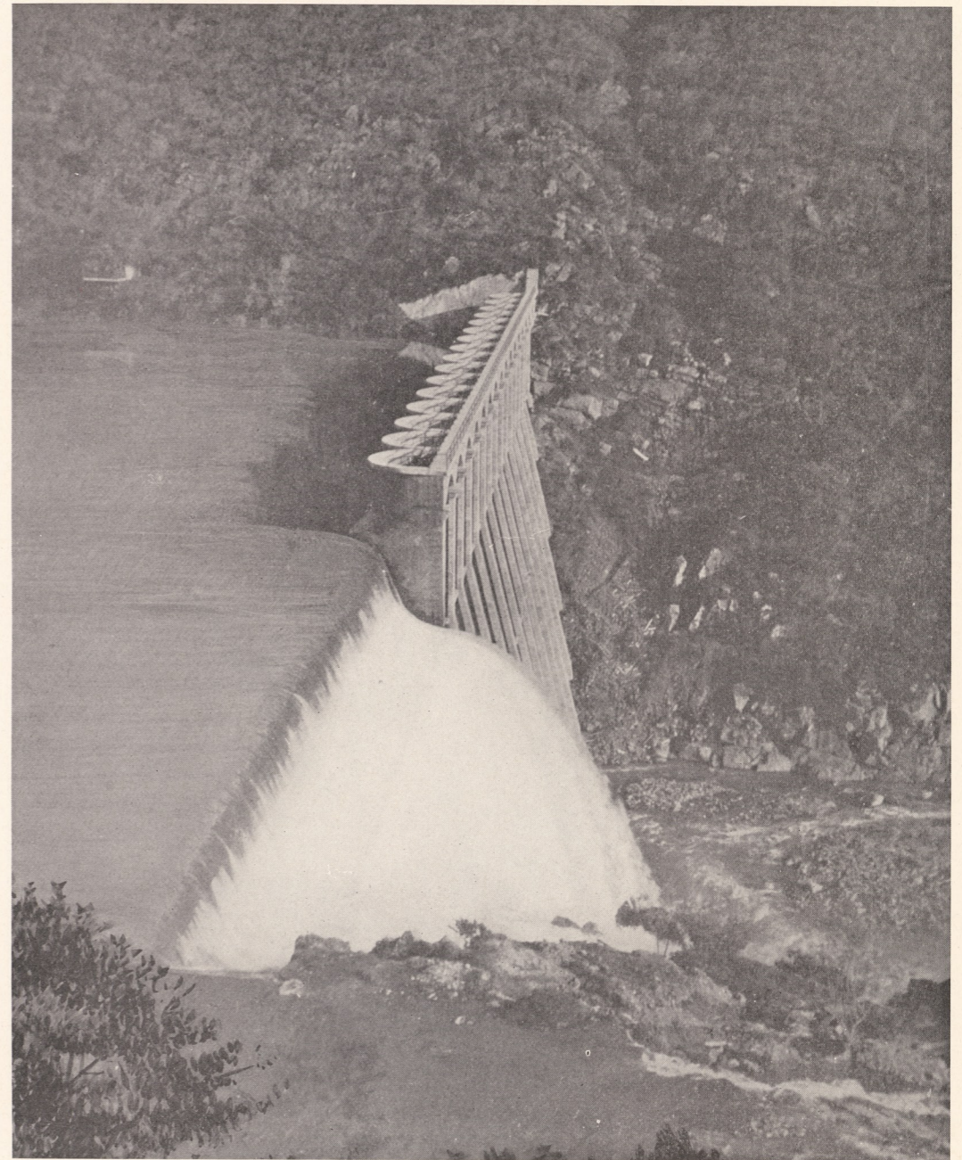
Lake Hodges Dam — 157 feet high; 750 feet wide.
