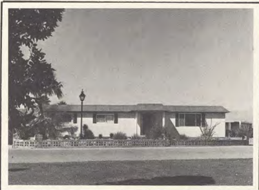
This mobile home is spacious and trouble-free, with a charming exterior and beautifully landscaped grounds.
