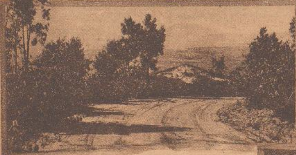
For months, crews of men have been at work laying out such roads as this one, following the contour of the rolling hills; taking advantage of natural scenic beauties.
