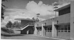
Detail of stairway to sun deck.
