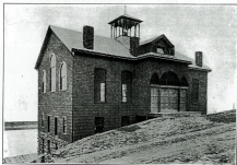
ROSETON'S ORNATE HALL AND CLUB BUILDING—PICK, PHOTOGRAPHER, NEWTOWN, N. Y.
