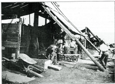
Brick Molding on Lynch Yards, Haverstraw, N.Y.*
