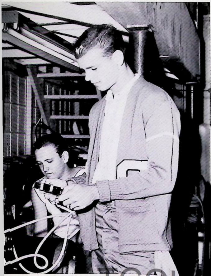
These students are learning the steps in building an air conditioning unit.
