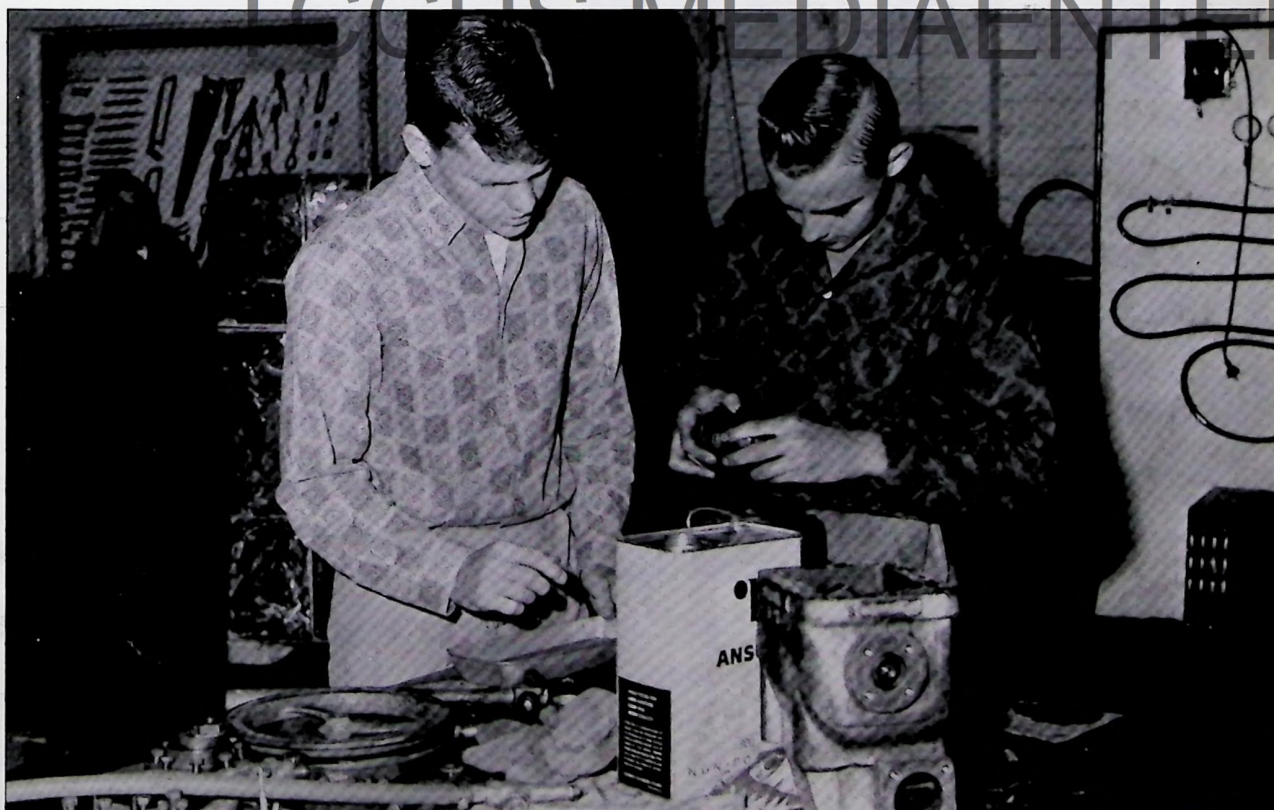
These boys learn how a compressor works by taking it apart.
