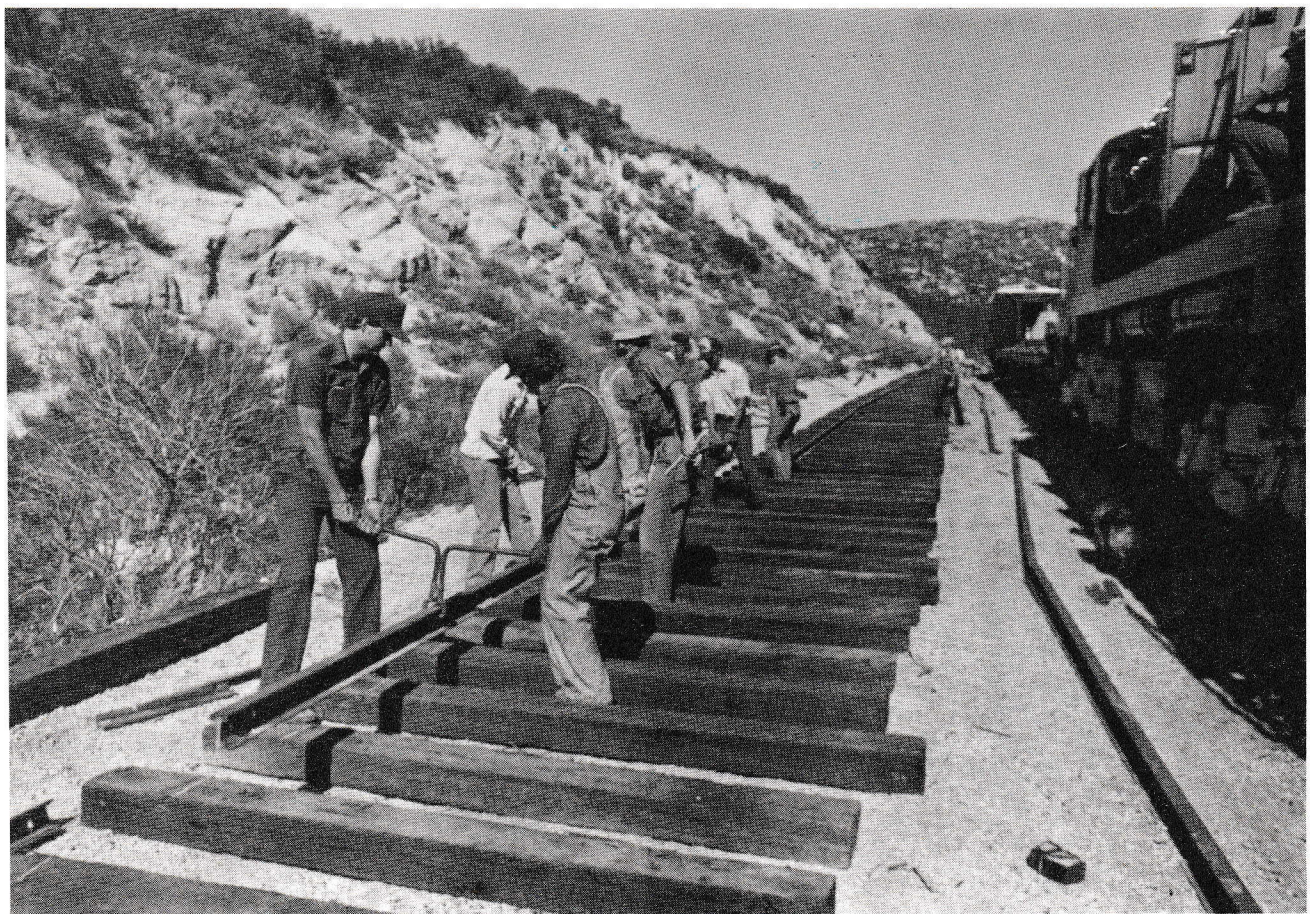
Rail is lifted onto the ties at our Clover Flat siding by an eight man crew who are (from front to rear) Jim Lundquist, Geoff Scheuerman, Jim Hamill, Charles Alban, Dick Ruppert, Paul Westover, Gaylen Dyreng and Ron Hyatt. Down the track, Dick Diestel and others spread joint bars, tie plates and spikes. L. Rose photo
