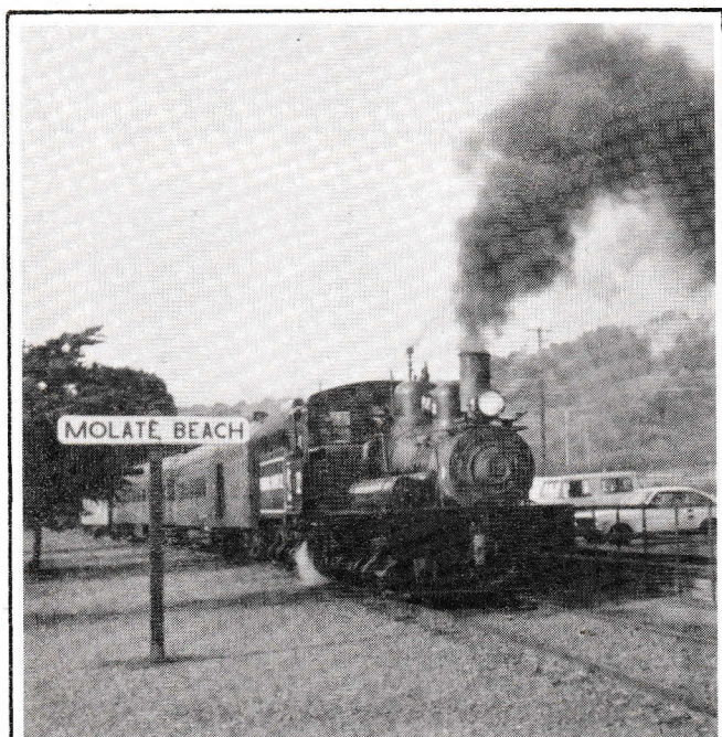
The Pacific Locomotive Association's Shay #12 hauls conventioners in nicely maintained Harri-man coaches at what was advertised as the last PLA steam up before having to move out of their Richmond facility. (L. Rose photo)
