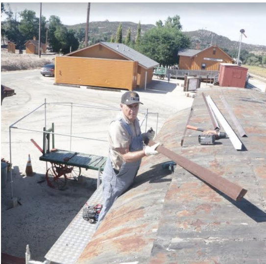
Left: Richard Finch reports progress on the Jacumba cars. The first half of the new fascia boards are finish and the install of them and the drip edge is in progress.
