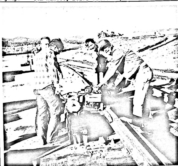
The rail saw bangs away on the point rails of switch #6 at the museum yard throat. Managing the machine are: (from left) Jim Hamill, Steve Oualline, and Cliff Pennick. Behind Cliff is a non member visitor who offered to help. (L. Rose photo)
