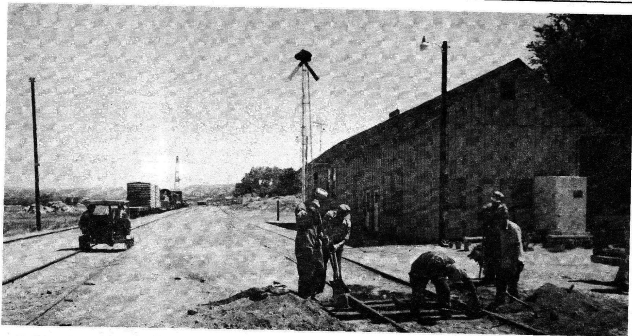
Trackwork on our SD&A is a never ending chore. The house track at the Campo Depot is a prime candidate for new ties. Shown here digging in new wood are (from left) Norm Heil , Gaylen Dyreng , Craig Coney , Geoff Shepherd and Floyd Lake . Other SD&A trackies have been Jim Lundquist , Charles Alban and Larry Rose . At left the fire speeder waits for the morning train to roll out of the museum grounds. (L. Rose photo)
