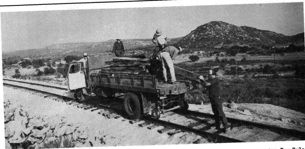
This high rail equipped dump bed truck has been loaned to the museum by railroad contractor Tom Pyle . It was promptly used to retrieve all the old ties, 400 in all, that we replaced on our SD&A this year. In this photo, from left, are Ron Hyatt, Joel Cox, Craig Coney, Charles Alban, and David DiGiorgio . A lot more ties can fit on this truck than a speeder trailer and it can be unloaded anywhere in seconds with just the push of a button. We expect this kind of action to be a regular chore each spring from now on as we labor to keep our much cherished railroad in top shape. The location shown is near milepost 68.5. (L. Rose photo)
