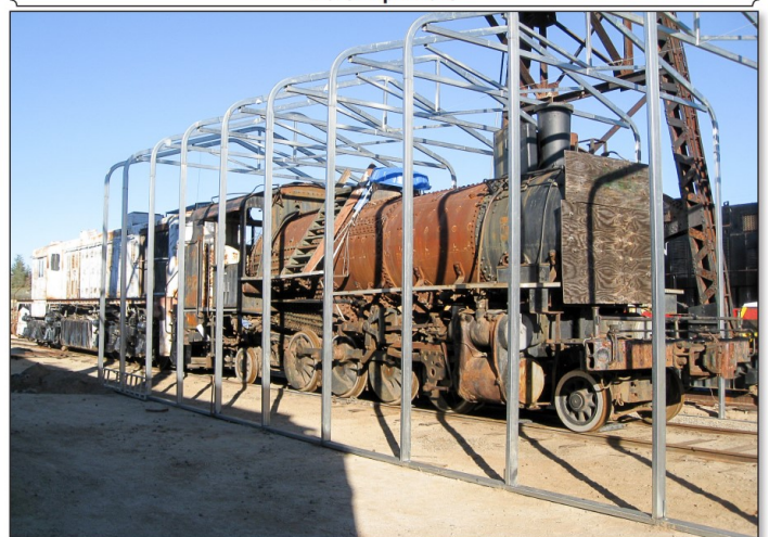
Progress is being made on the shelter for Coos Bay 11. All the frames are in place and the roof and side panels are being installed as weather permits. More pictures on Pages 4 and 5. Jim Baker
