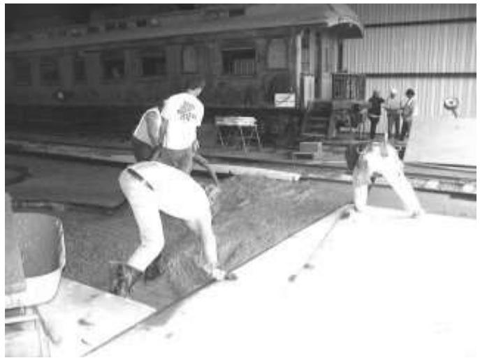
Concrete pour, phase #2 Ken Hansen photo
