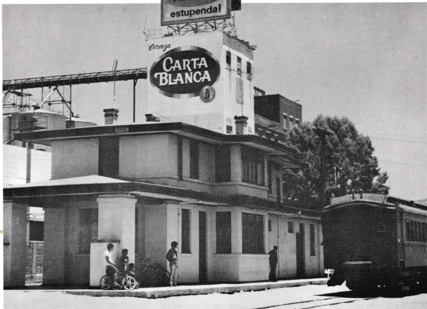
The main industry of Tecate is brewing beer. The brewery is the dominant structure of the town and is right behind the depot. This view of the station, built in 1919, is toward the northeast with SD&A coach #255 in front. For a similar view of this depot with nothing near it but a wooden water tank, see Bob Hanft's book "The SD&A, The Impossible Railroad", page 105. (Rene Scheuerman photo)
