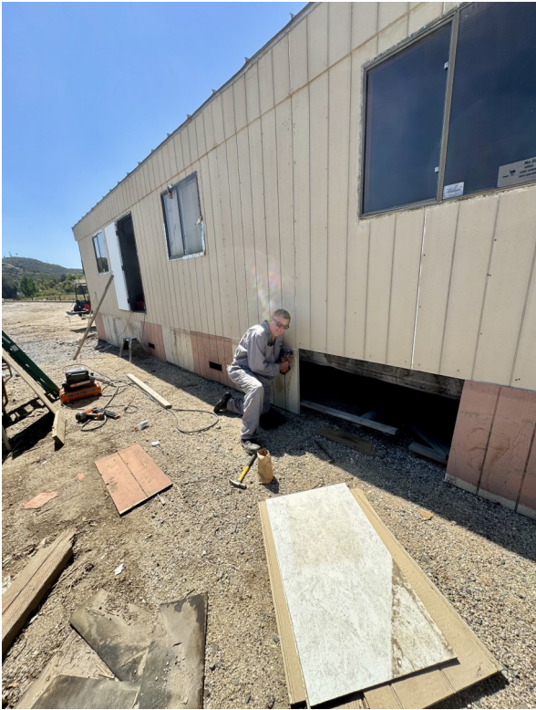
Jim Lundquist installs skirting on the office trailer
