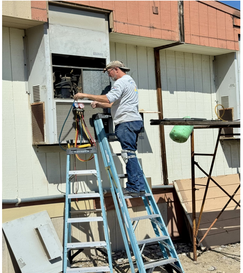
Air conditioning contractor services the units on the office trailer.
