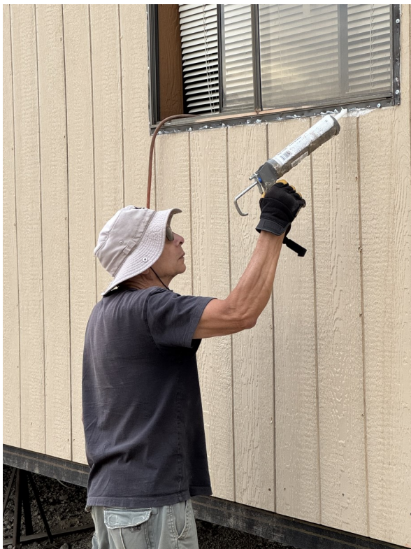
Steve Pohjola caulks windows on the Office trailer.
