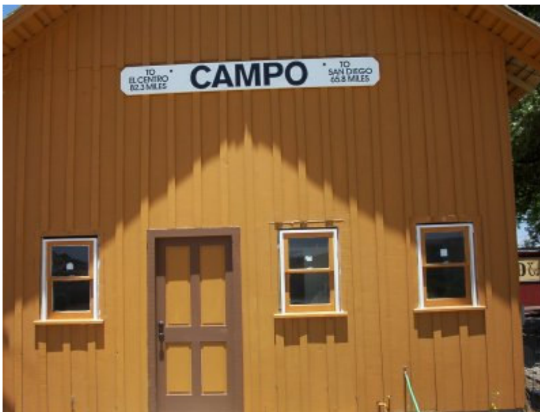
Three new windows mounted and looking good!
