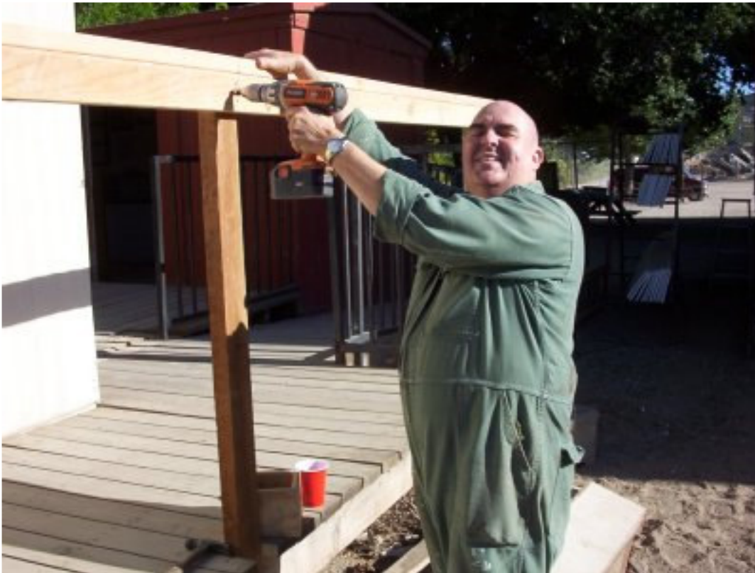
Larry Rose building a safety rail near the Campo Depot.
