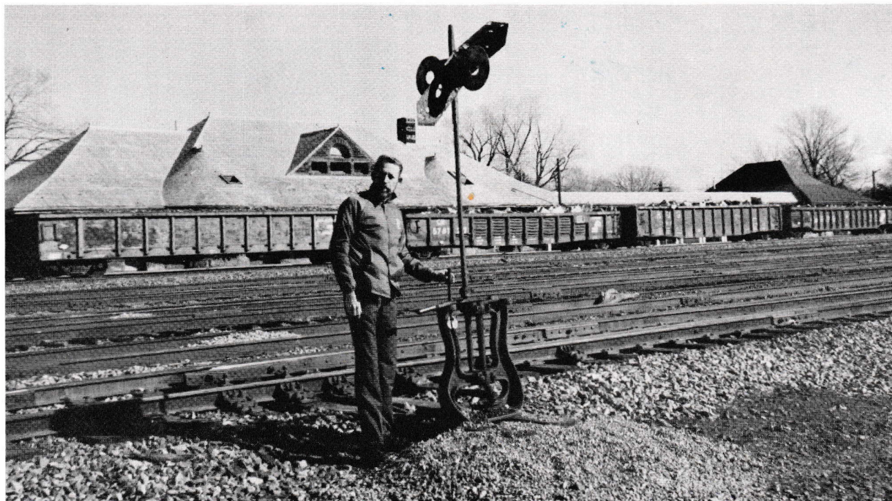
Museum Facilities Superintendant Barney Barnier inspects an unusual eastern style switchstand as a Conrail freight rumbles past the Sandusky Depot just beyond. The depot is boarded up and falling to ruin but Amtrak still stops here. The "agency" consists of a pay phone and bulletin board with the Amtrak schedule and reservations phone number. (L. Rose photo)
