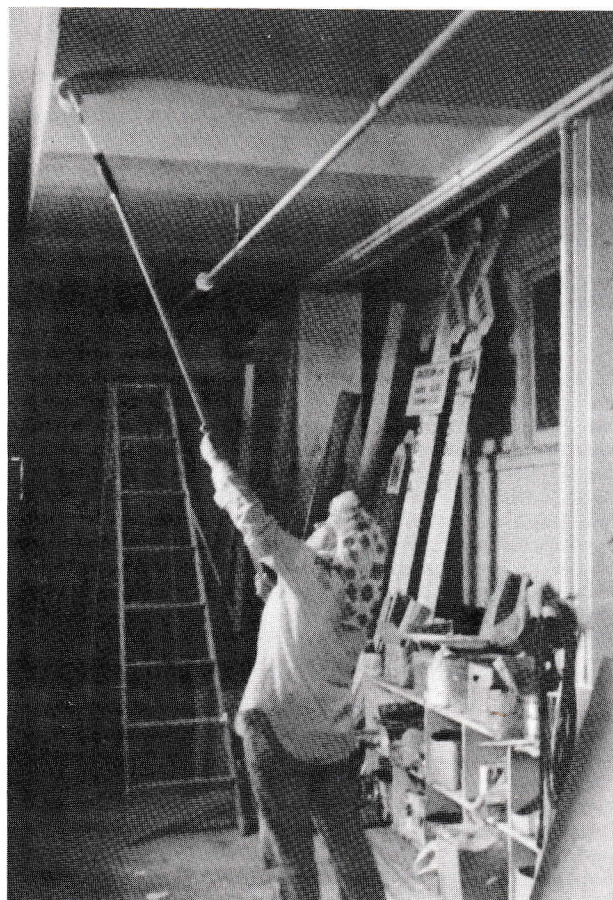
Tanya Rose is shown here painting the ceiling in the wood shop. Steve Wade did the carpentry to enclose the overhead. (L. Rose photo)
