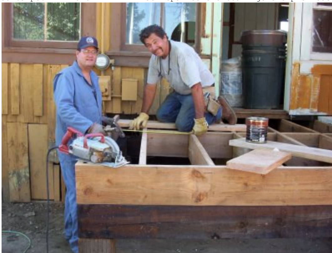
Jim Lundquist and Brian Elmore work on building a new giftshop entrance platform at the Campo Depot. Randy Houk photo.
