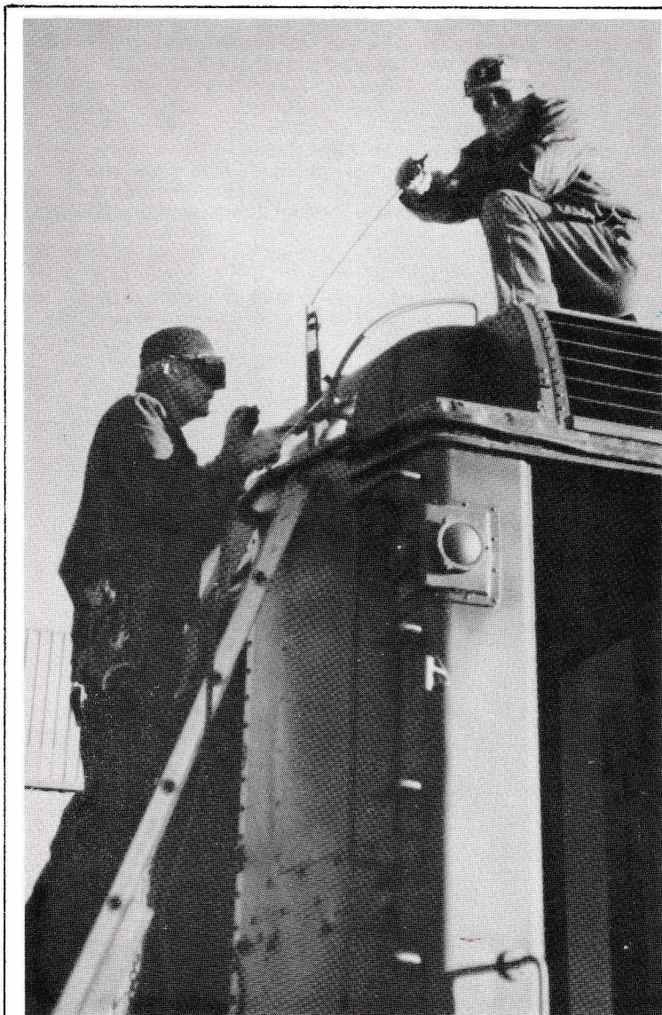
Here is Dick McIntyre, on ladder, and Paul Bortell repairing the sheet metal roof of S.D. & A. coach #253. Paul, on the car roof, is using a special sheet metal bending tool designed and built by Dick just to work on the ends of the clerestory roofs of these ex-Lackawanna veterans of 1925. (L. Rose photo)
