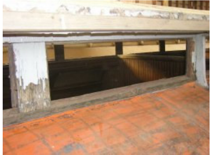
Clerestory progress on the Jim Crow car.
