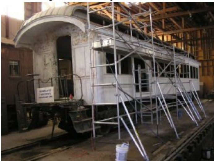
Scaffolding assists in work on the Jim Crow car in the car barn.
