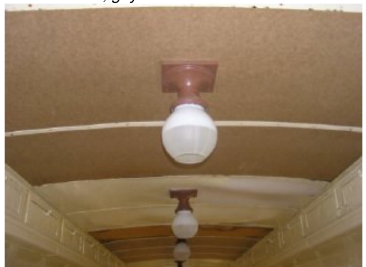
New ceiling panels replace rain-damaged ones in SD&A coach #252!
