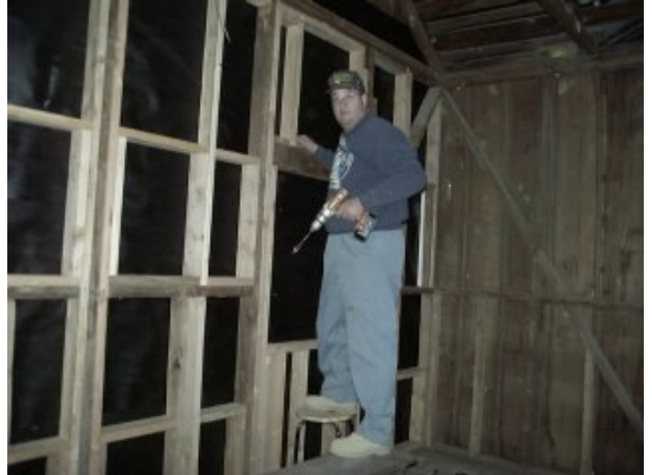
Jim Lundquist works on window framing. Ken Hansen photo
