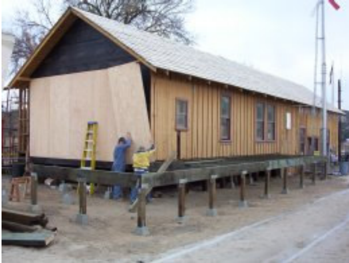
Jim Lundquist & Bill Armfield install plywood siding.
