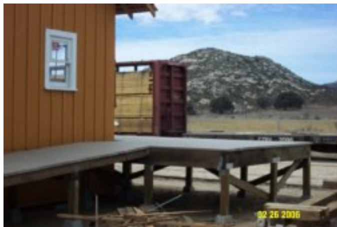
Platform and ramp nearing completion. Steve Spiker photo
