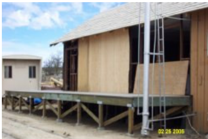
Trackside depot and platform progress. Steve Spiker photo
