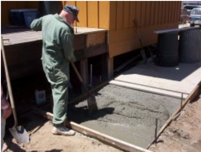
Larry Rose prepares a concrete footing at the depot.
