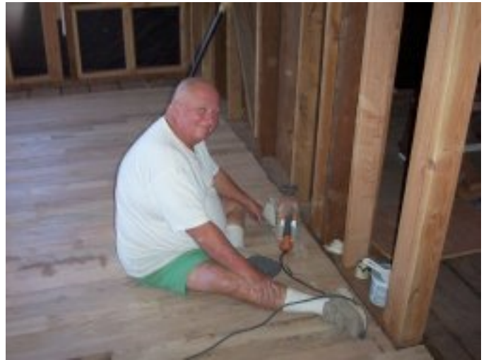
John Little works on the new floor upstairs.
