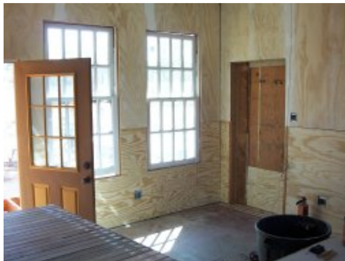
Inside the new baggage room
