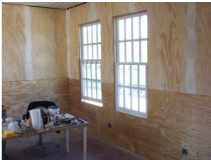
Inside the new baggage room
