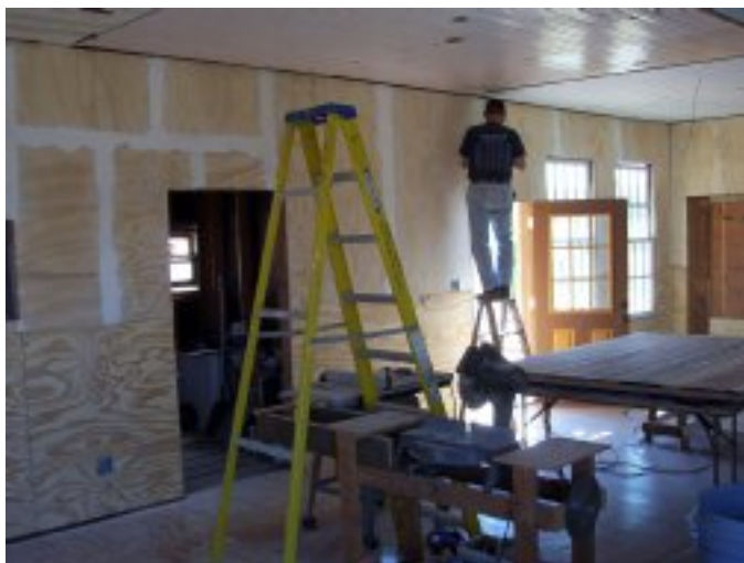
Inside the new baggage room
