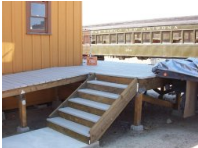
New steps to the loading platform
