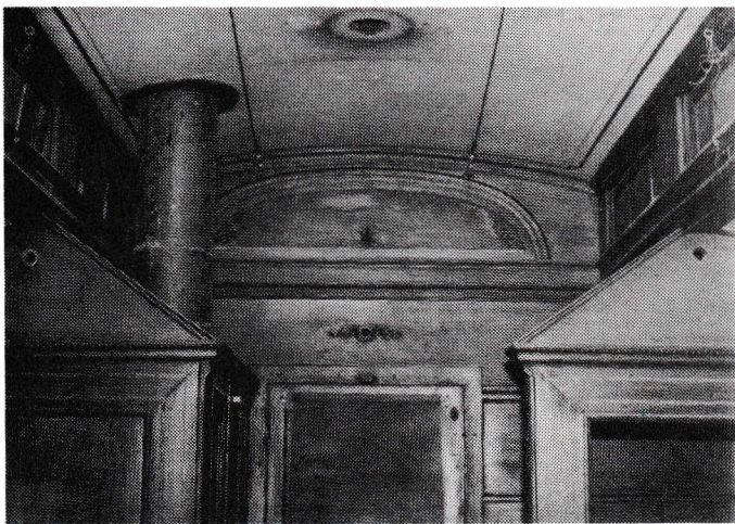
Forward end of D&R #14, shows details of restroom roof (left) and alcove (right) where there may have been a stove in pre-D&R days. Note the ceiling wires, which may have been installed by 20th Century Fox when the car's oil lamps were removed.
