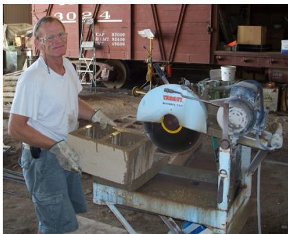
Red Schmitz cutting concrete blocks for the pit
