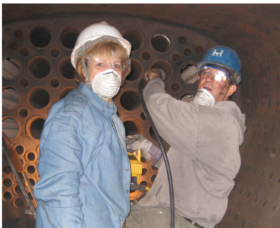
Linda Corvan and Mike Lucek cutting flues in the firebox
