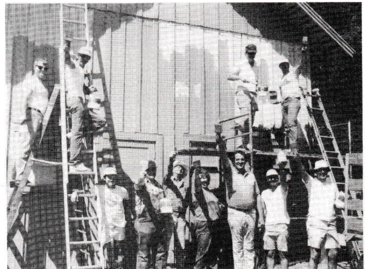
This is the crew that gave the Campo Depot a badly-needed coat of paint last month. Not only did they have a great time working together, but were treated afterward to a super spaghetti dinner by Maxine Sanborn.
