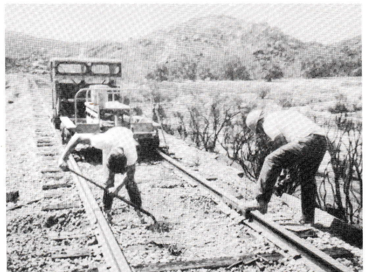
Brett Burrell and Rick Borstadt cutting in ties replacing those burnt during a brush fire around Milepost 64, October, 1989.
