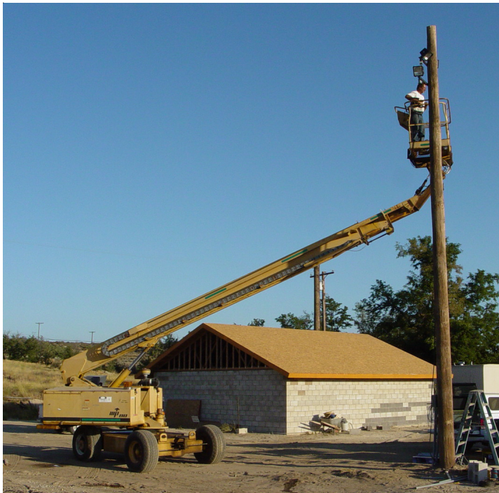
Brian Elmore in the cherry picker mounting a bank of four flood lights.
