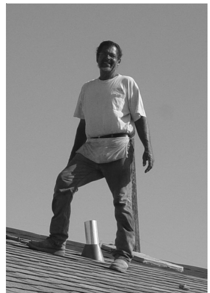
Brian Elmore works on putting shingles on the new toilet building down by the depot
