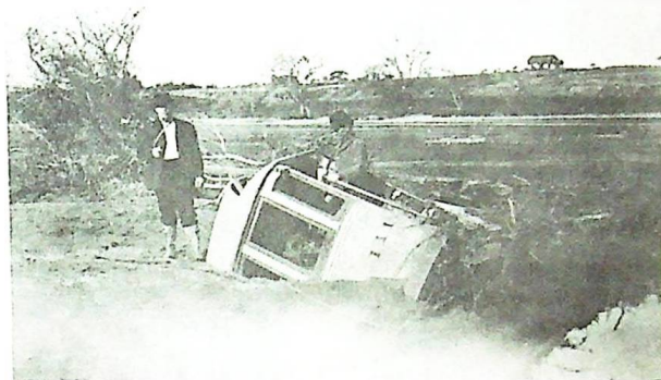
San Diego & South Eastern Railway Combo #111 buried in debris of Sweetwater Valley flood, 1916. Car was demolished. (R. P. Middlebrook)
