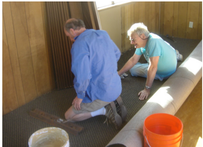
Bruce and Bob installing new carpet in the Library Trailer
