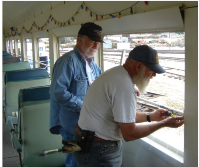
Frank and Don installing windows
