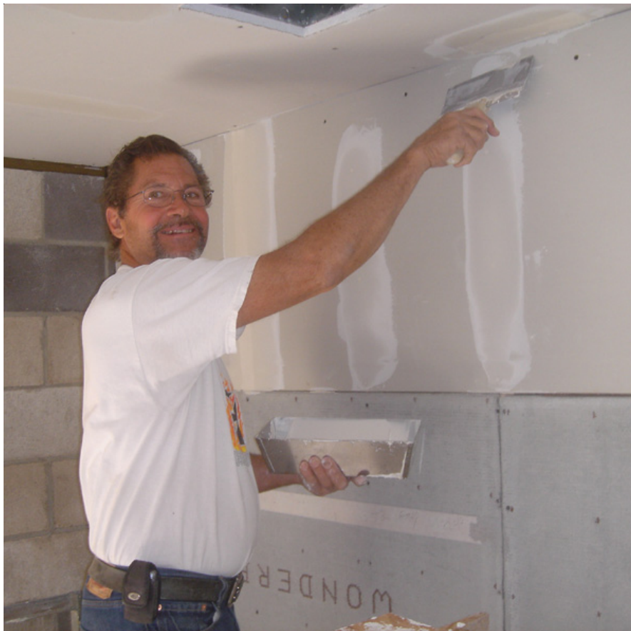
Brian Elmore filling in the drywall gaps in the new restroom
