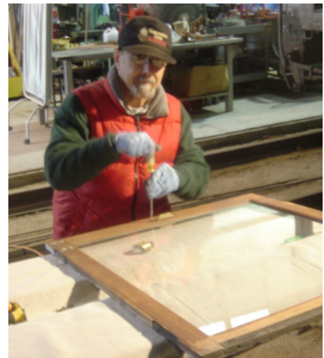
Ted putting the latch hardware back on a completed window
