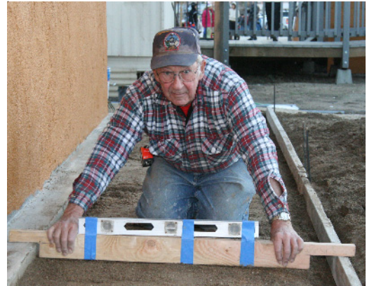
Bill Armfield preparing the bathroom walkway Photo by Frank Denison
