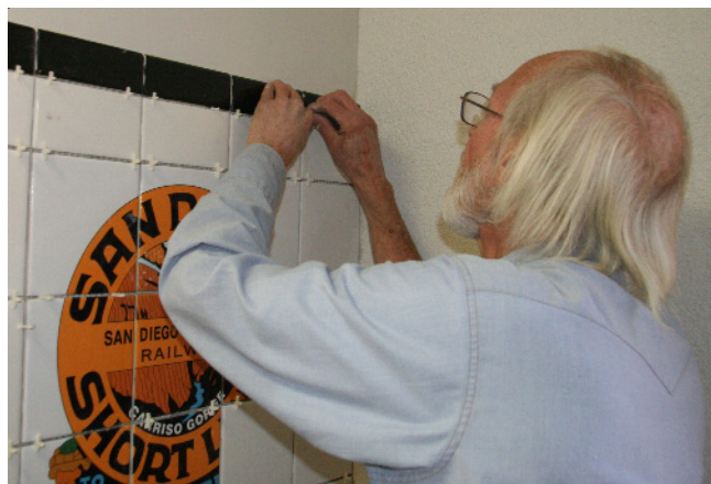
A volunteer tiles in the new restroom
