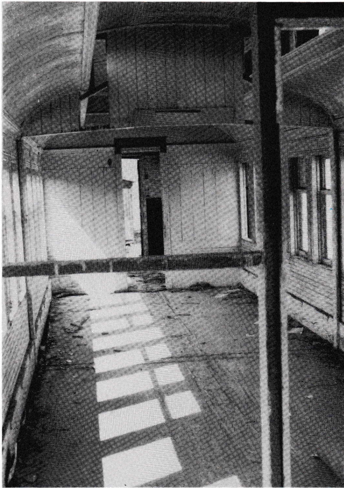
Interior view of the one-time Garcia quarters showing the original smoking-section partition and the remains of two temporary walls. photo-w.niedrich
