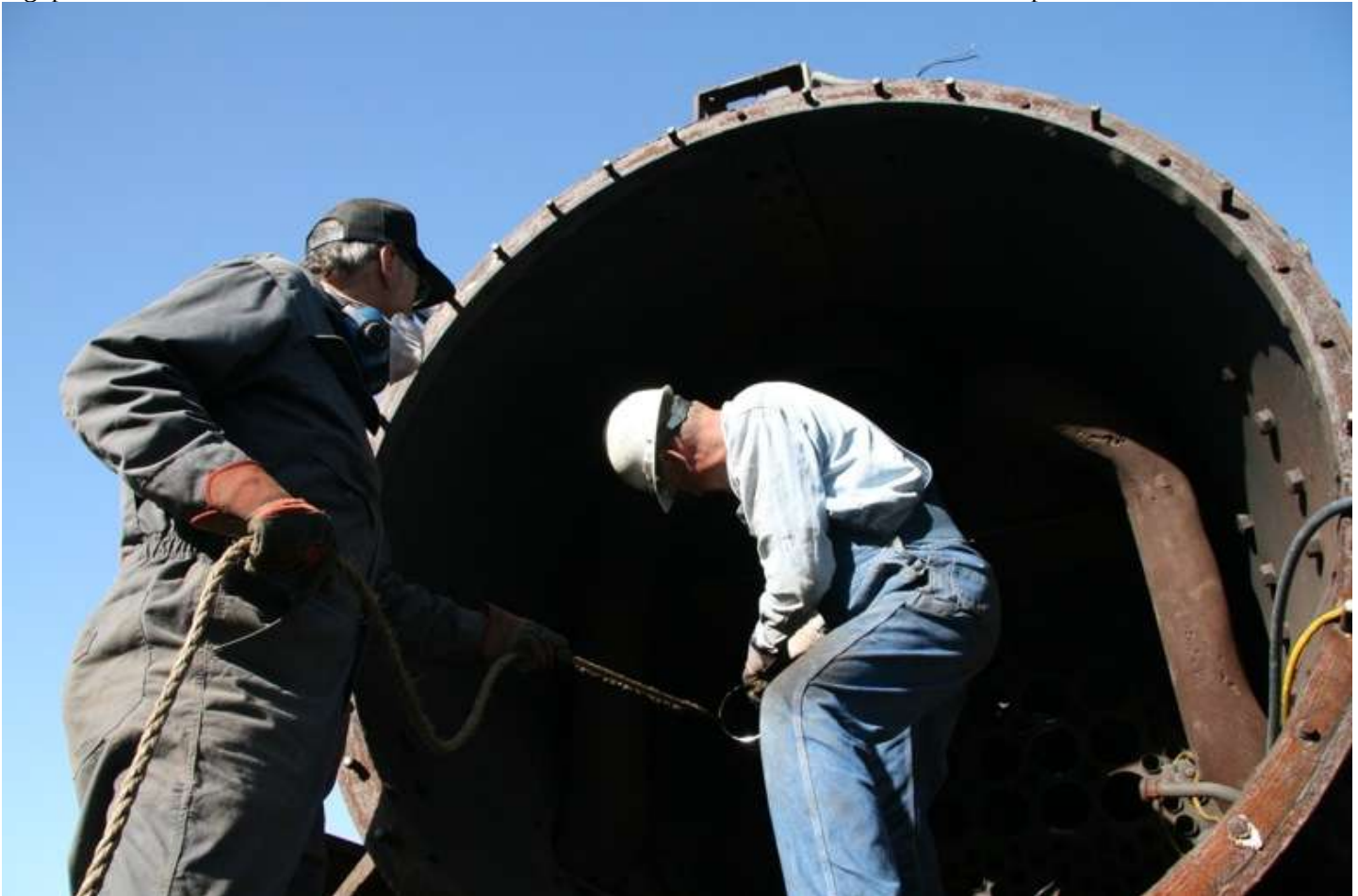
Here are Bob Nickles and Rich Paulus working in the smoke box cleaning the blasting sand
