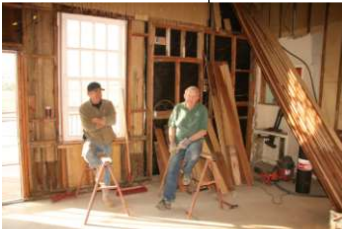
Ken Hanson and Bill Armfield take a break from removing the interior wall boards. In the rear can be seen the old framing for a window taken out by SP in the 1960's. This window will be put back in. In the corner is the semaphore operating levers that will remain.
