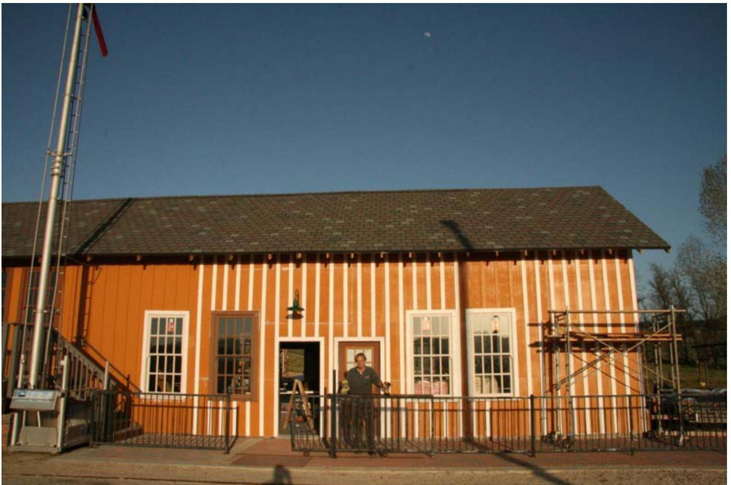
John Shannon late in the day on April 24th as he finishes the batts on the NW (or track side) of the Campo depot. All the windows are new, custom-built to match the 1916 vintage originals and placed in the original locations. Frank Denison Photo
