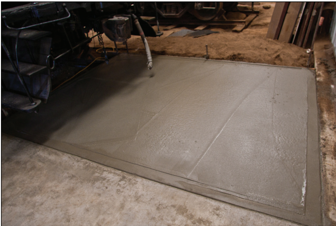
The concrete pad poured at the west end of the Jim Crow Car #3. John Wright Photo
