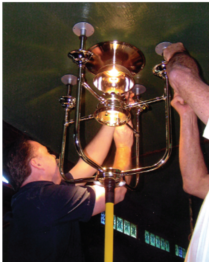
Woody installs one of the lamps in the Jim Crow car. Frank Stites Photo
