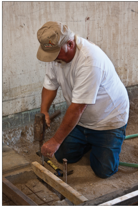
Don Getz builds forms in the car shop. John Wright Photo
