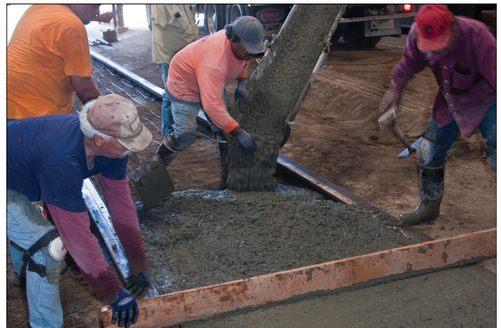
From Left to Right: Robert Rangle, Joe Ringe, Jose Rangle and Americo Yescas pour concrete in the shop. John Wright Photo
