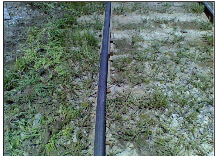
A close-up of the weed crop. The weeds growing in the ballast are particularly hard to get out, sometimes yielding only to pulling out by hand. There is still a lot of moisture in the cut; the decomposed granite is damp just under the surface.
