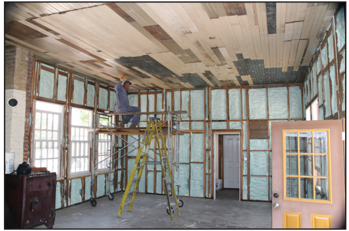
Jim Lundquist at work on the depot ceiling. All the exterior walls are now insulated. Frank Denison Photo
