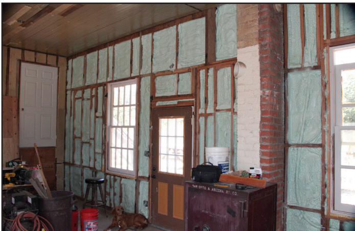
The new insulation can be seen in the unfinished exterior walls. Frank Denison Photo
