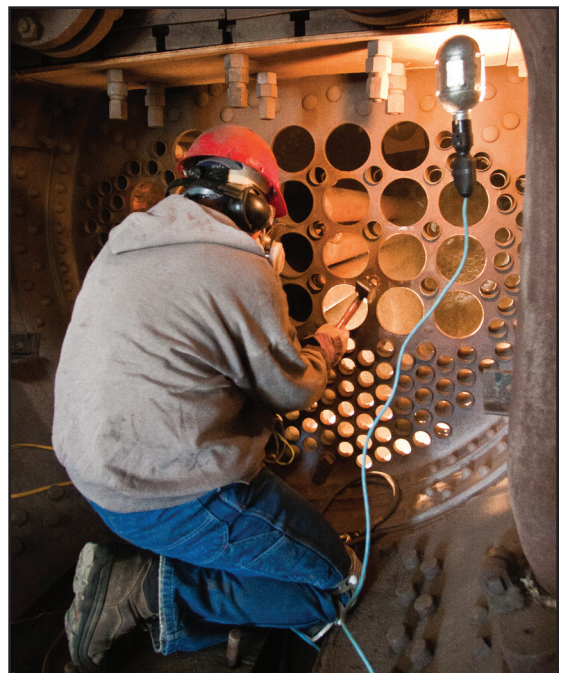
Mike Lucek attempts to remove a boiler tube stub from Coos Bay No. 11. John Wright Photo
