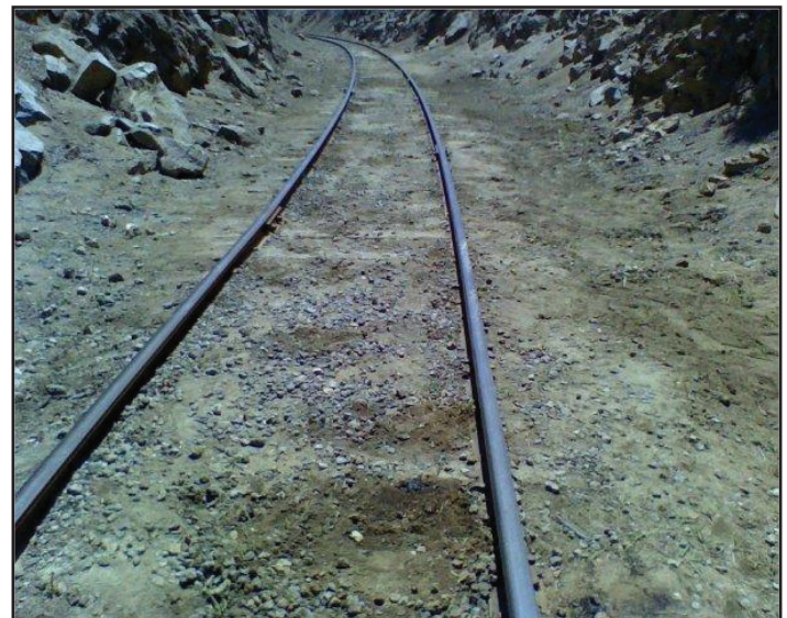
Looking west, the right-of-way has been cleared.
