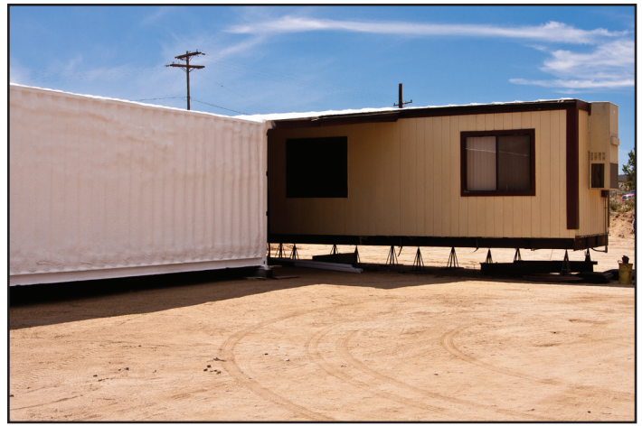
The library trailer is complete and the storage containers have been covered with insulating foam and reflective paint.
