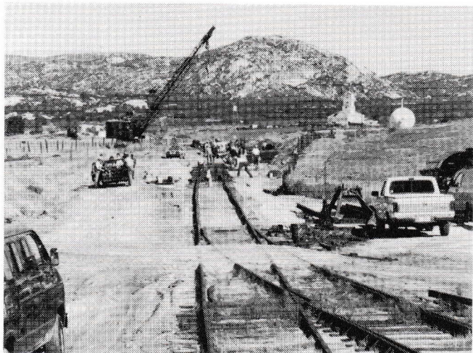
Looking northeast up the east lead toward its connection to the SD&IV main line, 35 to 40 Museum volunteers are working all along the quarter-mile stretch of new track.
