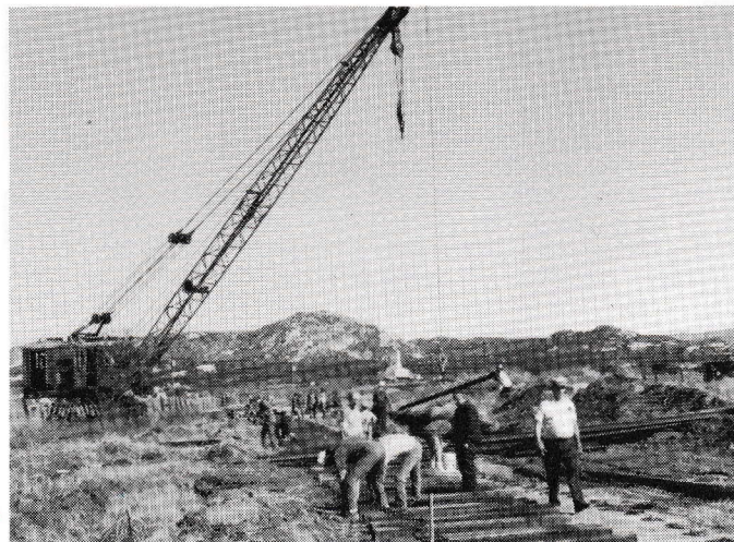
SDRM volunteers laying track on the east lead into the Museum yard. Our ex-Navy self-propelled crane is working from the SD&IV main line.
